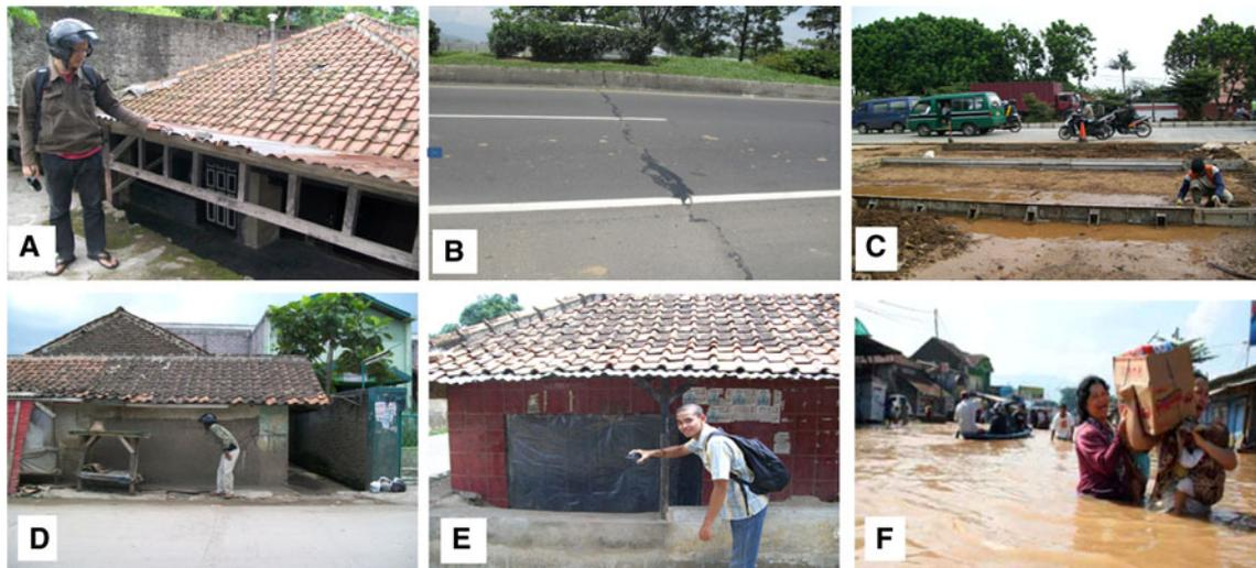
**Fig. 4** Examples of recent subsidence features in the Bandung Basin. Photos taken by Irwan Gumilar in 2010. **a** Subsided house in the Dayeuh Kolot area (around DHYK GPS stations); **b** highway cracking in the southern Cimahi area (around CMHI GPS station); **c** uplifting of the road due to subsidence in the Gedebage area (around
